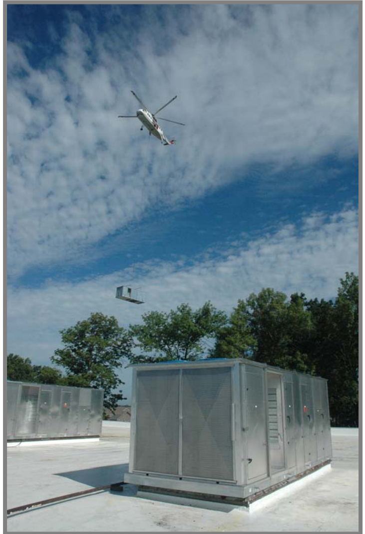
Helicopter setting one of ten units on rooftop of high school. (Two of the ten units were set by crane.)
