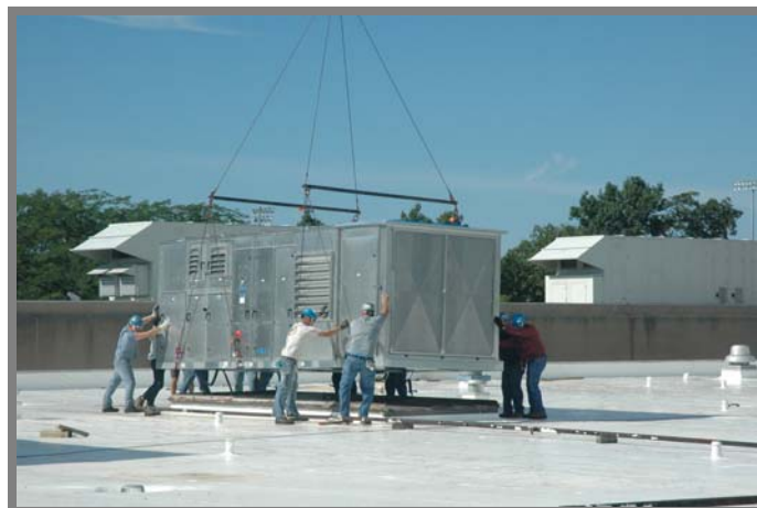
Helicopter setting one of ten units on rooftop of high school. (Two of the ten units were set by crane.)
